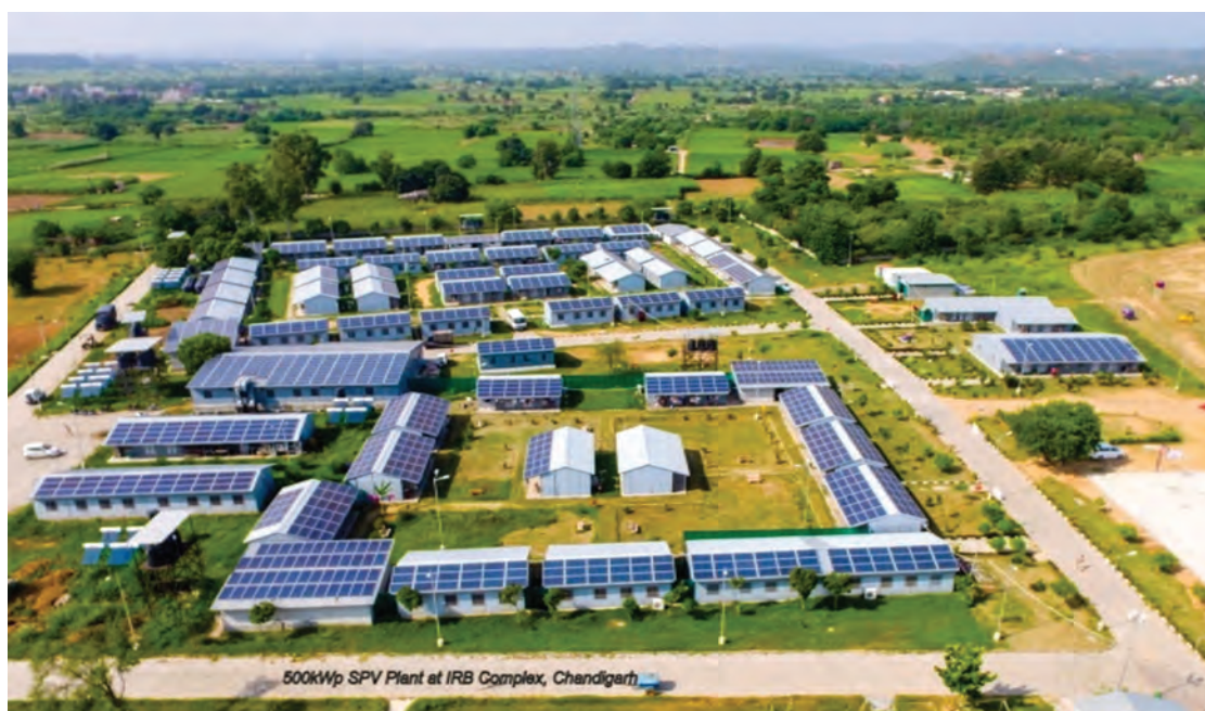
Figure 75: 500kWp SPV Plant at IRB Complex, Chandigarh
