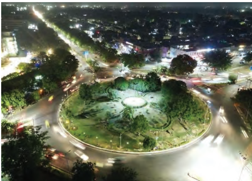
Figure 59: Roads and Street Lighting having LEDs in Chandigarh
