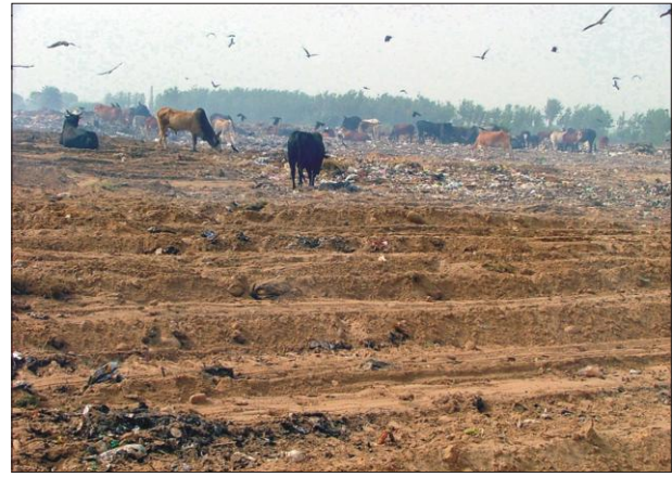
Present Dumping Ground with partial compaction
