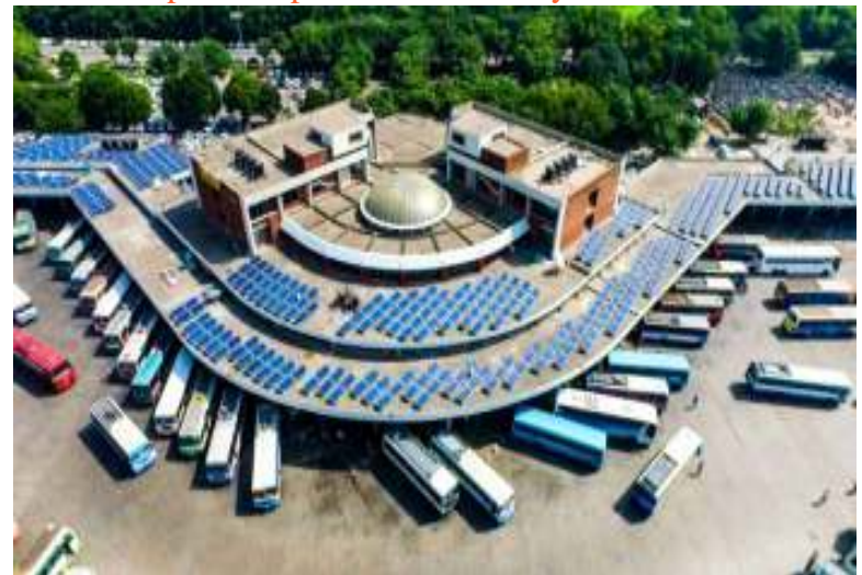
200 kWp Rooftop Solar Plant at ISBT, Sec-43
