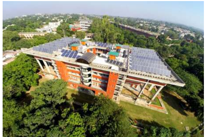
50 kWp Rooftop SPV Plant at Paryavaran Bhawan
